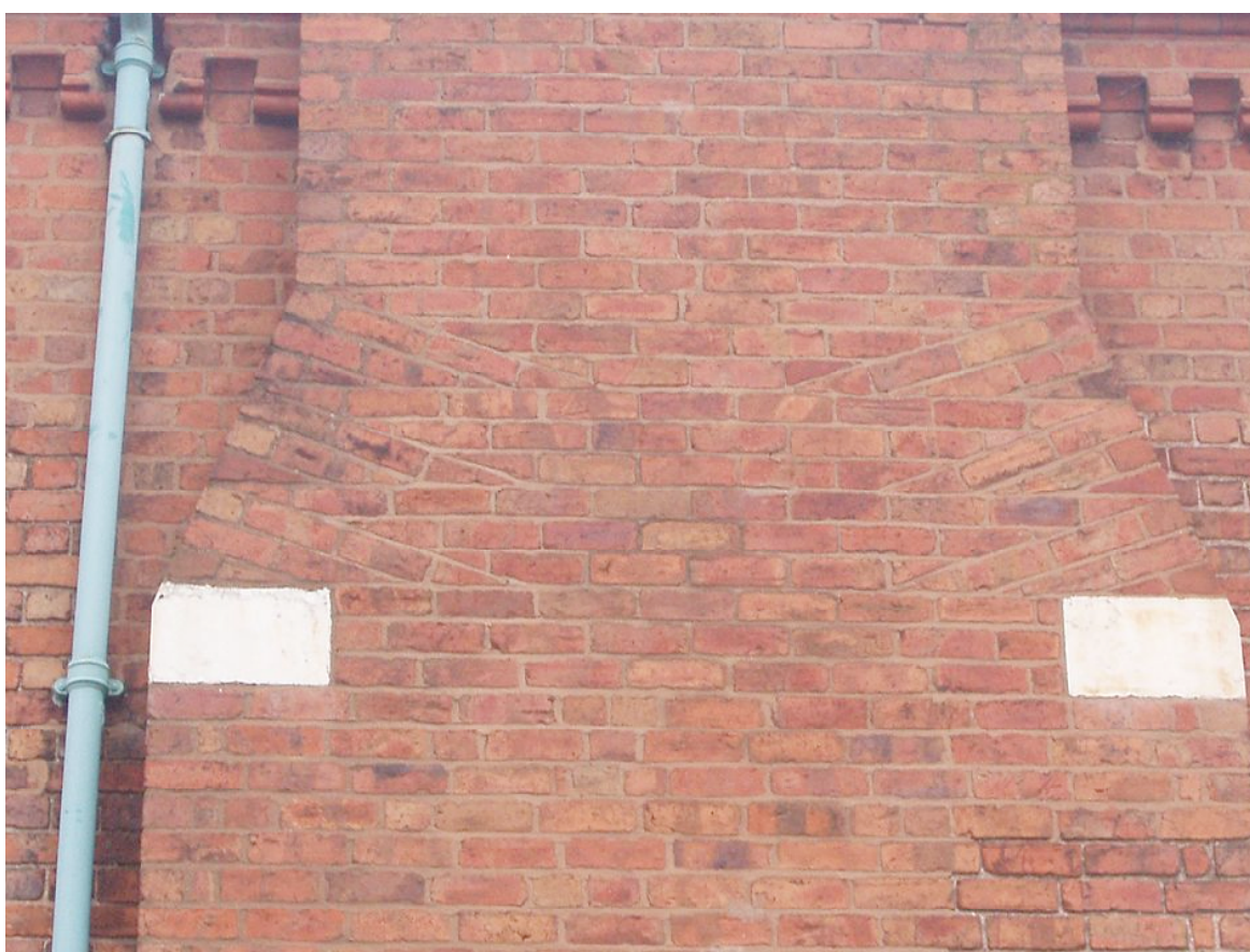
Fancy brickwork in the Chimney of this building. Keith Shaw September 2007
