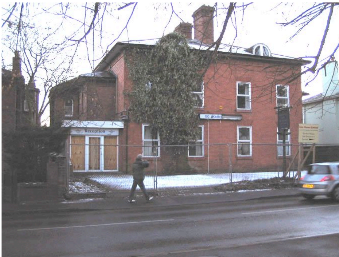
194 & 195 Comberton Road prior to demolition Nicky Griffiths 1st March 2006
