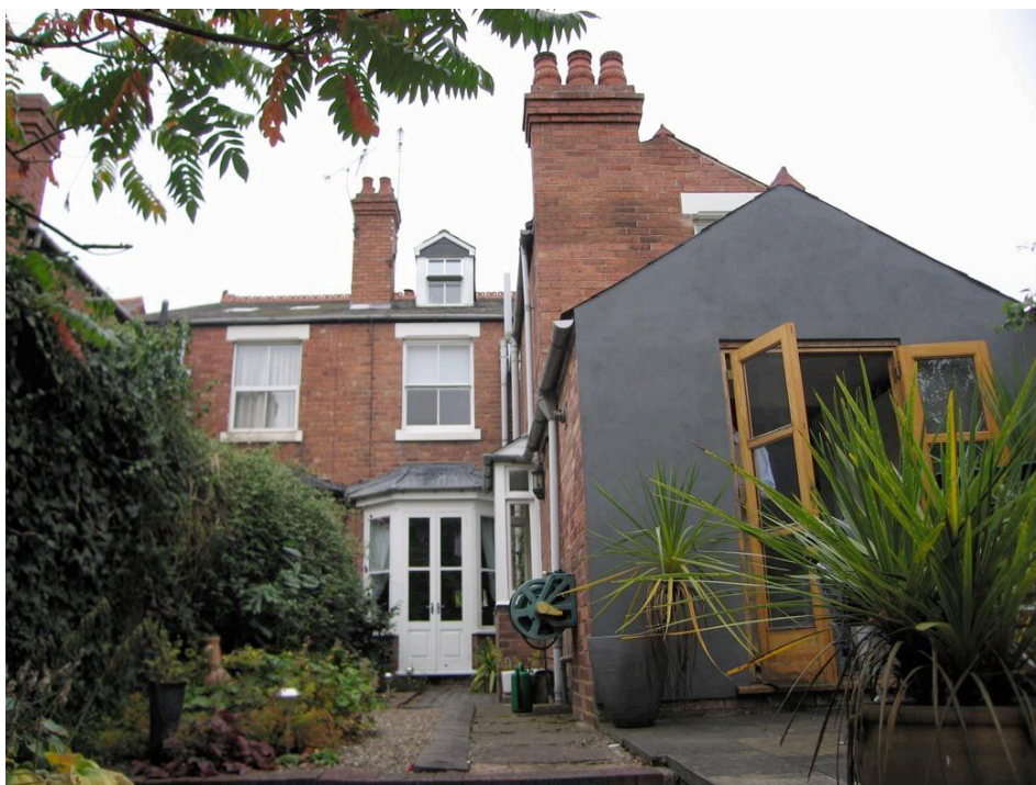
Rear of number 47 showing the substantial rear extension
