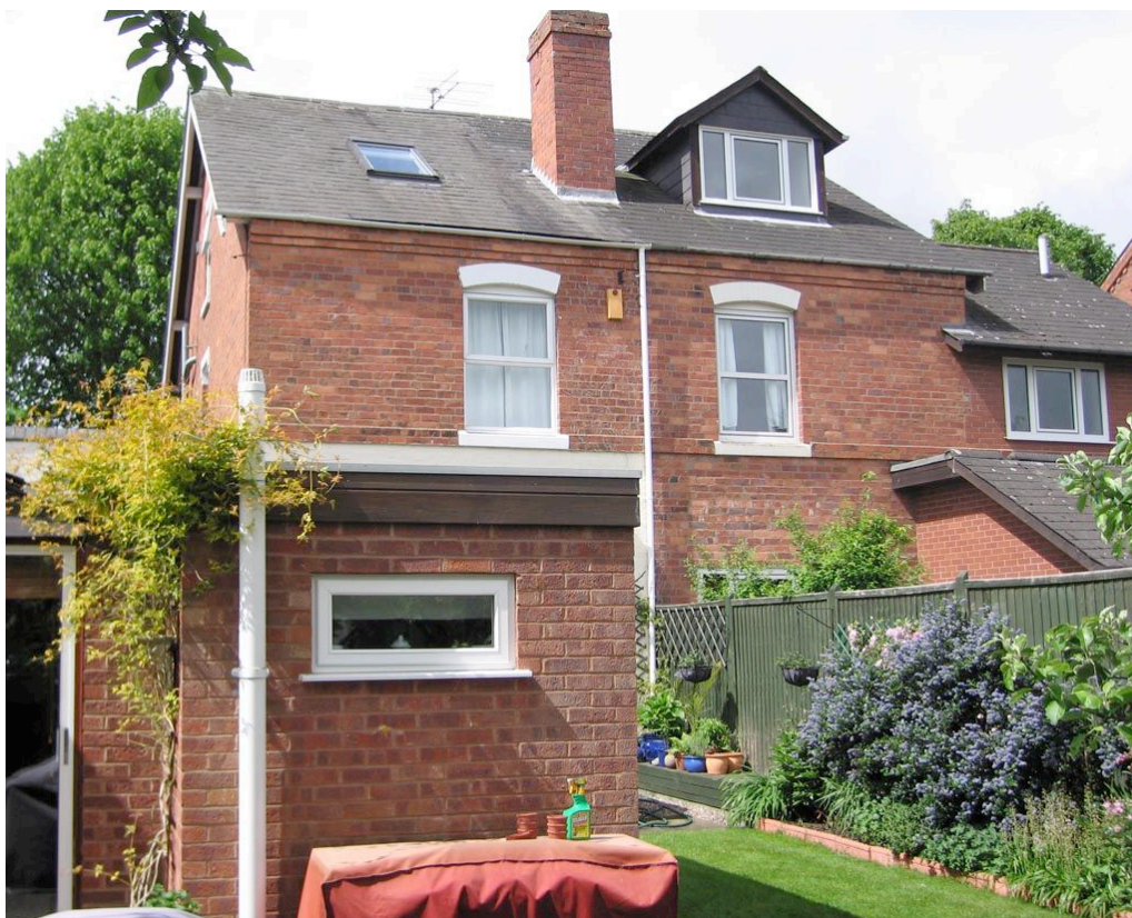
Rear of house in 2007
