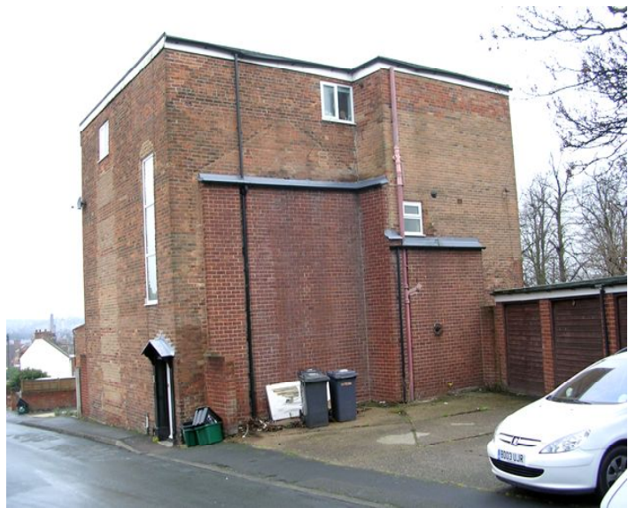
Fig. 3(b) Looking West
