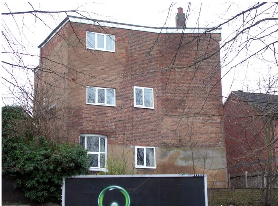
Fig. 3(c) Looking South from Coventry Street
