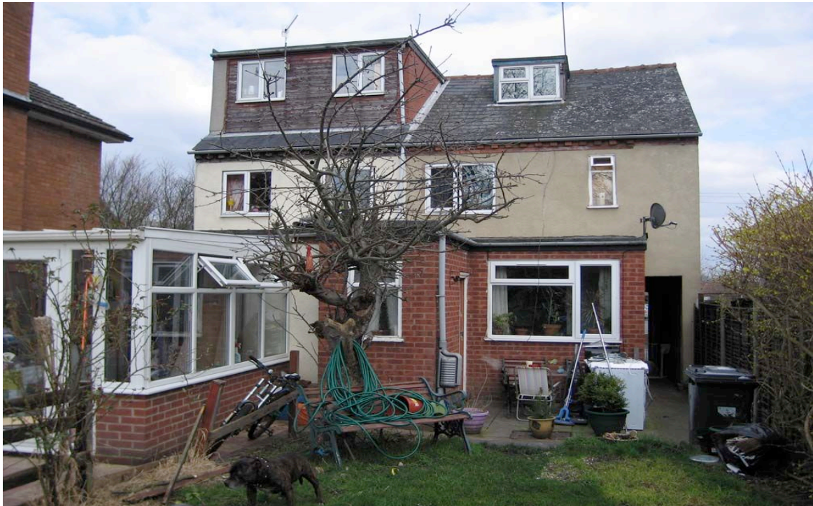
Rear of the two houses
