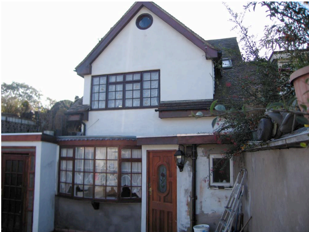
5 Woodward Road transformed - pictured in 2007
